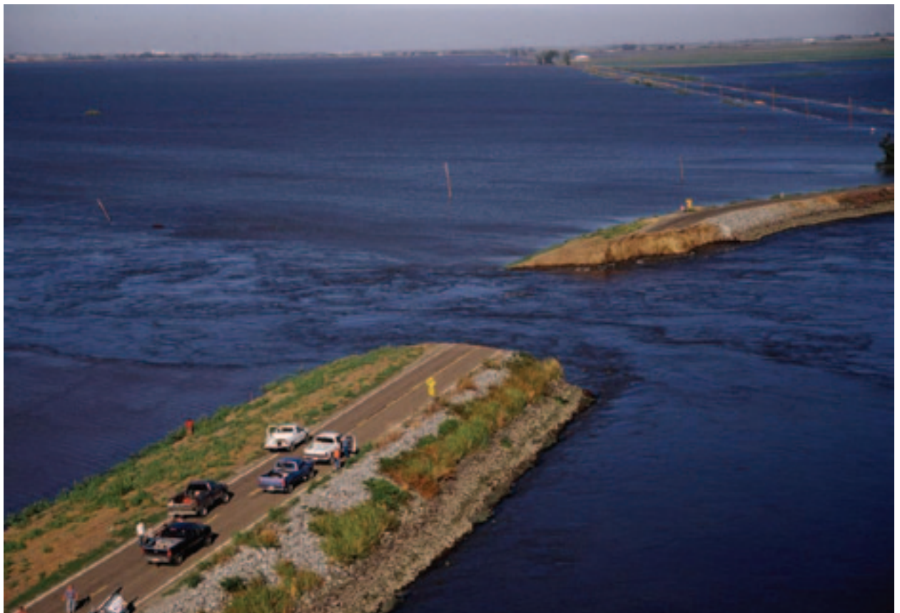
Levee Failure
