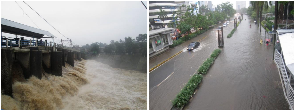
Figure 1. The outlet of the Upper Ciliwung River at the Katulampa weir (for location see Figure 2), south of Bogor city, West Java, Indonesia in January 2014. (left picture, source: https://commons.wikimedia.org/wiki/File:Bendung_Katulampa_Januari_2014.jpg ) Peak flow as observed here could arrive in the city of Jakarta in about half a day, causing severe flooding. (right picture, source https://www.flickr.com/photos/budiwins/8391569698/ )
