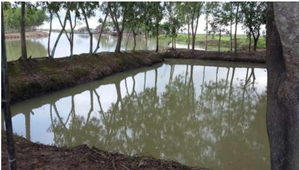
Rainwater harvesting pond at the Auk Ka Ba sluice gate site
