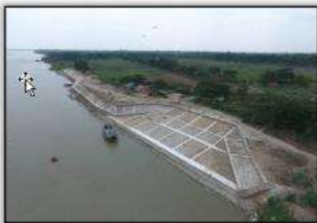
River banks protection works
