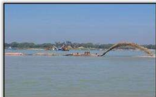
River dredging works
