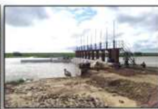
Sluice Gates by IWUMD(ID)
