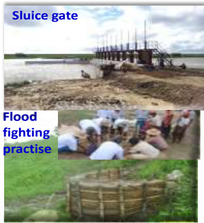
Flood protection works
