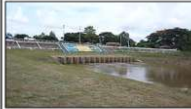
Mezali Sluice Gate
