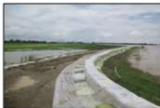
Flood protection embankments by IWUMD (ID)
