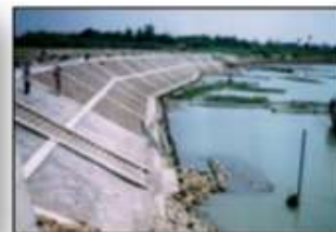
River bank protection works by DWIR
