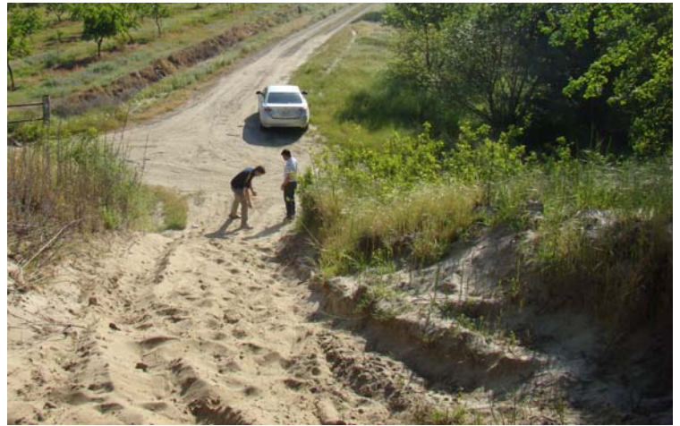
FIGURE 10: Backside of Antiquated Sand Levee.
