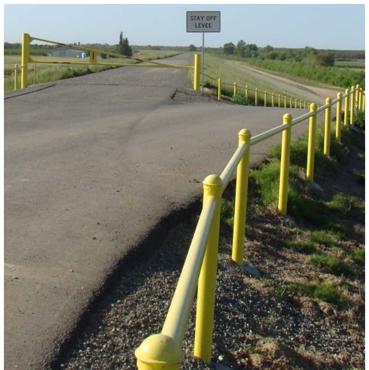
FIGURE 11: New Setback Levee after Completion.
