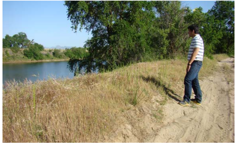
FIGURE 9: Feather River & Antiquated Primary Levee.
