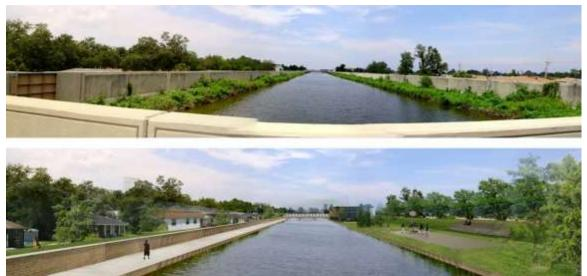
Figure 19 Outfall canal New Orleans – existing situation (top) and impression of the future situation (bottom). Source: Dutch Dialogues.
